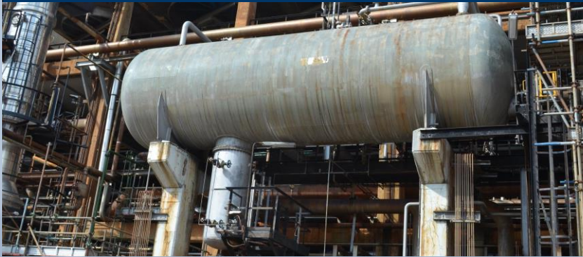
The Main Column Top Accumulator in the Main Fractionator Overhead System is a three phase, horizontal separator that separates condensed Crude Main Fractionator overhead from sour water and hydrocarbon vapour. This vessel is equipped with a water boot that facilitates phase separation.
