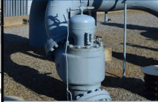
Crosby Style JOS Pressure Relief Valve Figure F2-3
